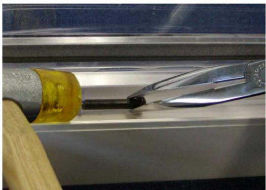
5.) Catch the hinge- pin with the pliers and pull; if necessary hit the pliers with a rubber mallet.
